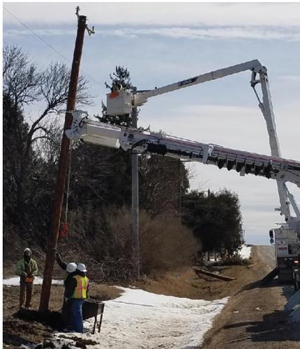
*Grundy County REC lineman building a new line to replace the old underbuild on ITC's line. Karl Nielson is in the bucket, while Eric Freese is using the ground controls. Tony Sienknecht and Aaron Bird are lending a helping hand.*
