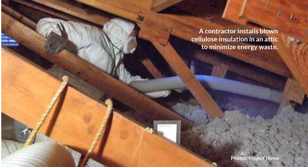
A contractor installs blown cellulose insulation in an attic to minimize energy waste.
