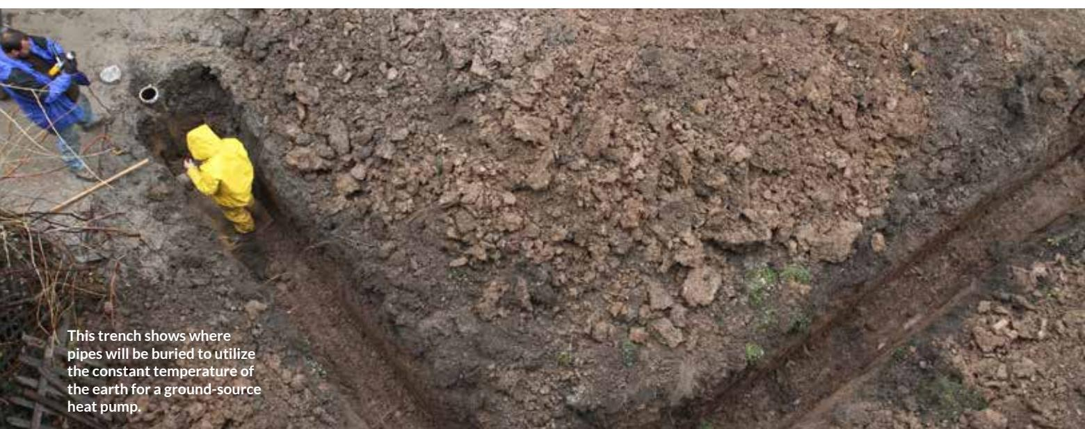
This trench shows where pipes will be buried to utilize the constant temperature of the earth for a ground-source heat pump.
